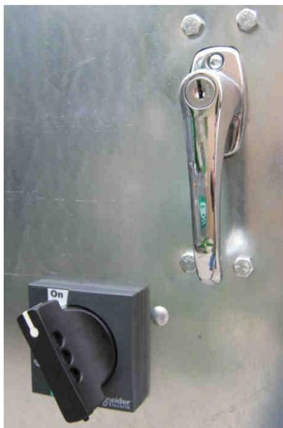
Image 10 – Latch and Main Disconnect switch in “On” position
