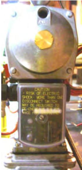
2ND GAS VALVE ACTUATOR WITH REGULATOR
