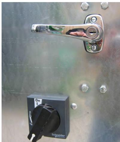
Image 2 – Door latch and Main Disconnect switch
