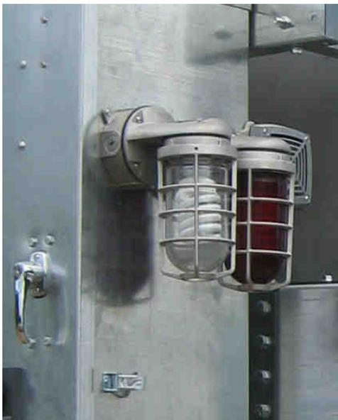
Image 19 shows work light, alarm light and alarm buzzer.
