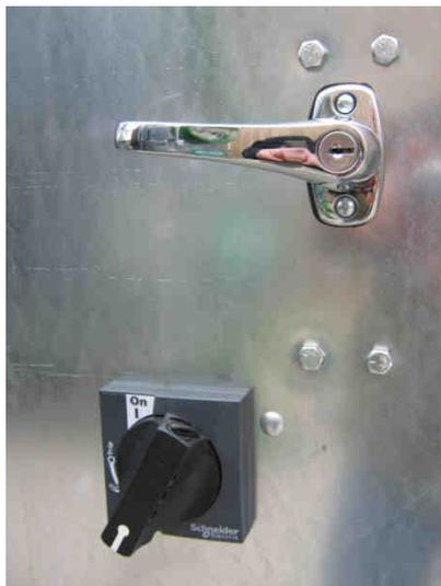
Image 9 – Latch and Main Disconnect switch in “Off” position
